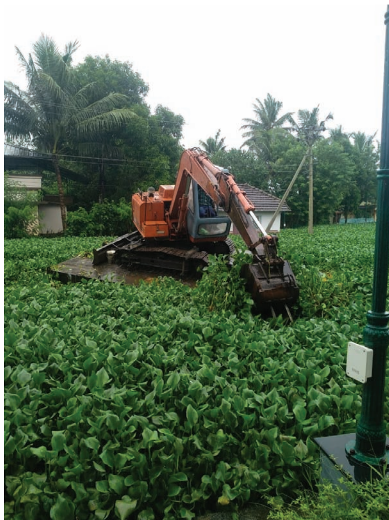
Figure 26 Mechanical removal of water weeds in progress, Kuttanad, 2019 Source: Department of Water Resources.
