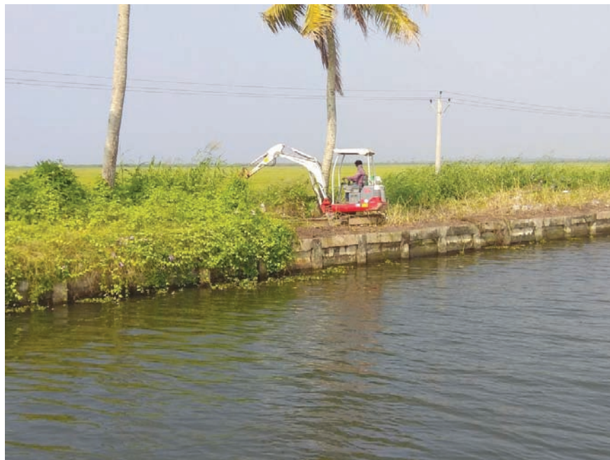
Figure 16 Outer bunds of kayal padasekharams completed using the pile and slab method, Kainakari North, Kuttanad.
