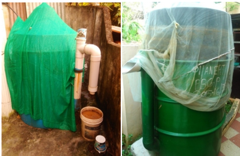
Picture 4.3.3 & 4.3.4: Biogas Plants Covered with Net by the Beneficiary to Prevent Mosquito Growth
