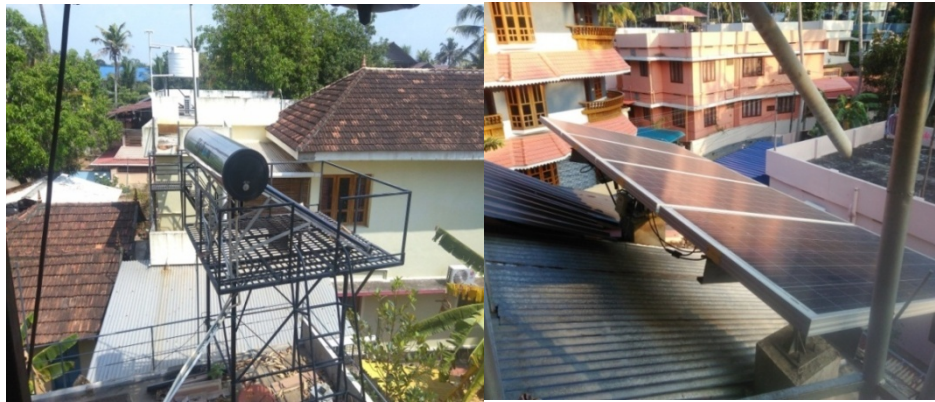
Picture 5.6 & 5.7 Additional Structures for Solar Panels and Solar Water Heater Erected by Mr. Jeevan
