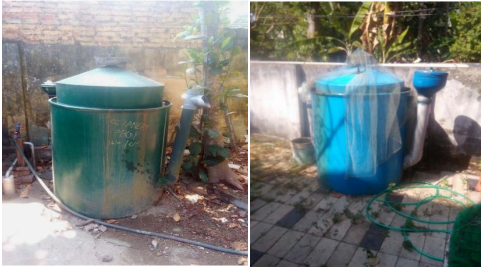
Picture 4.3.7 & 4.3.8: Malfunctioned Biogas Plants due to Improper Waste Dumping
