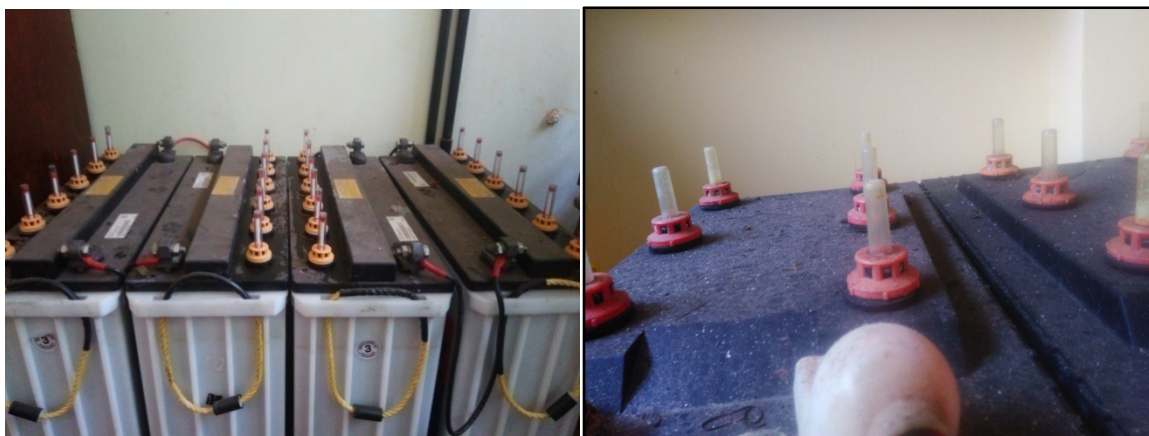
Picture 4.3.23 & 4.3.24: Batteries which are Properly and Not Properly Refilled with Battery Water
