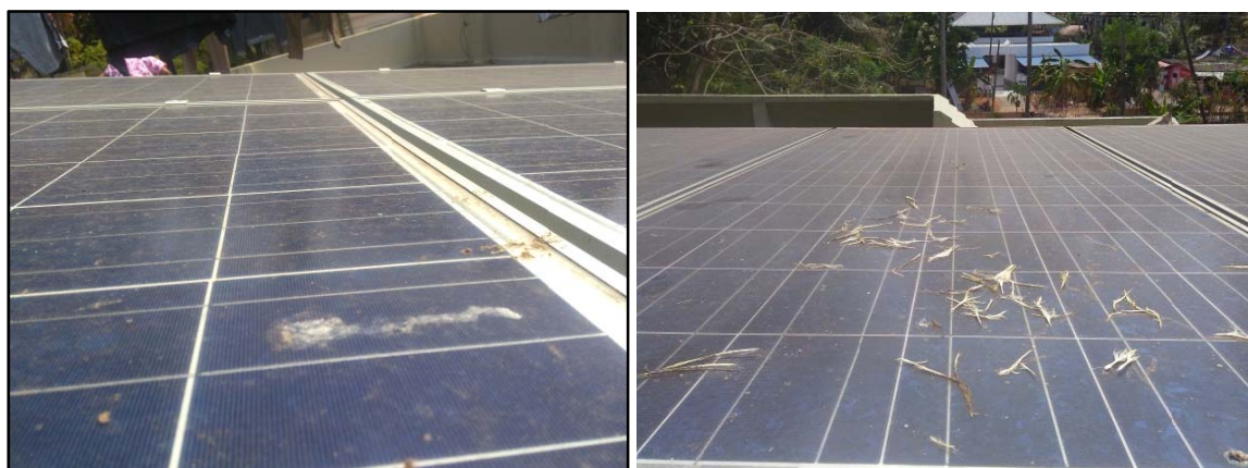
Picture 4.3.21 & 4.3.22: Solar Panels which are Not Properly Maintained by the Beneficiaries
