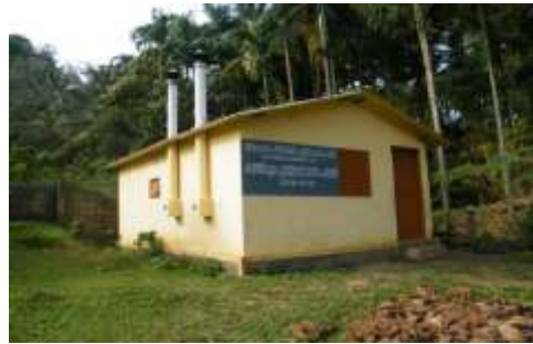
Renovation of kitchen in Kakkuppady LPS
