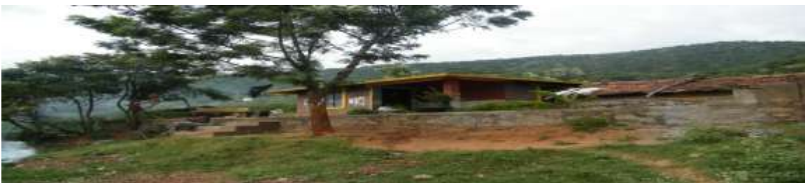
THDP in progress: A success story of AHADS initiative
