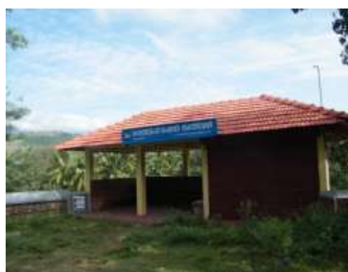
Waiting shed: Bhoothivazhi
