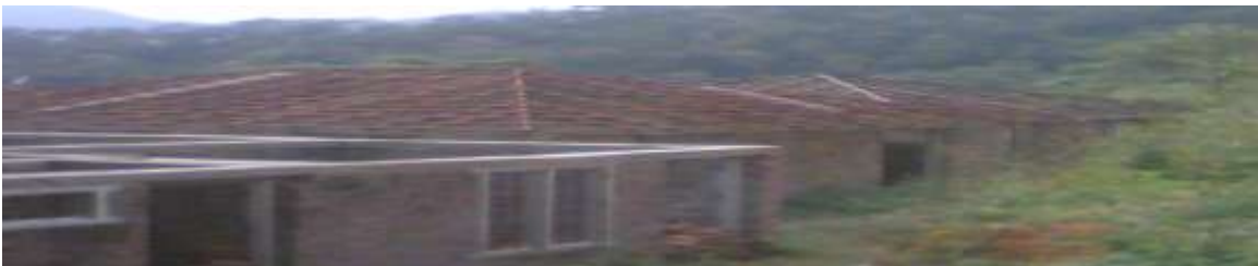
THDP in progress
