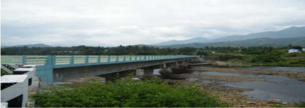
A view of Chavadiyur bridge: AHADS initiative
