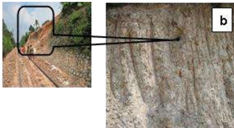
**Fig. 4.2:** Mulathuruthi railway cutting where a section of the laterite cutting failed
