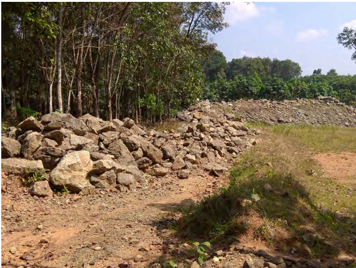
Figure 14 Rocks and rubble dumped on the alignment of the Edayar Distributary in the MVIP
