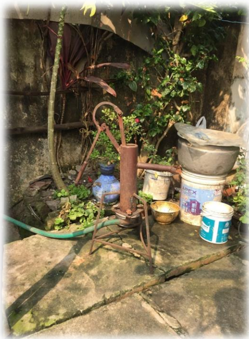
Plate 5.6 Rusted Hand Pump adjacent to drainage
