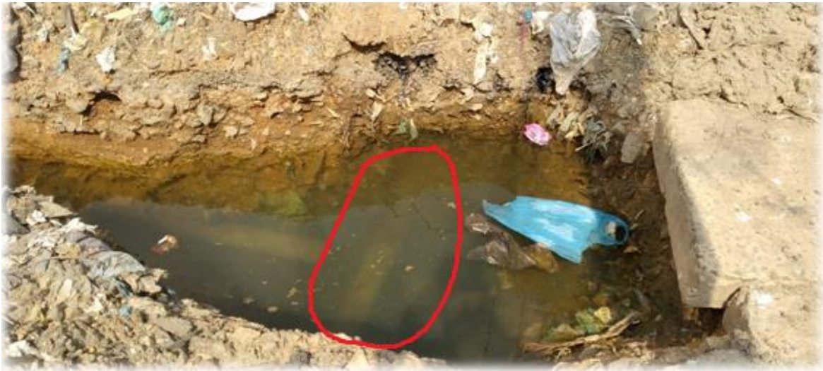
Plate 5.6 Domestic Pipeline connection through drainage
